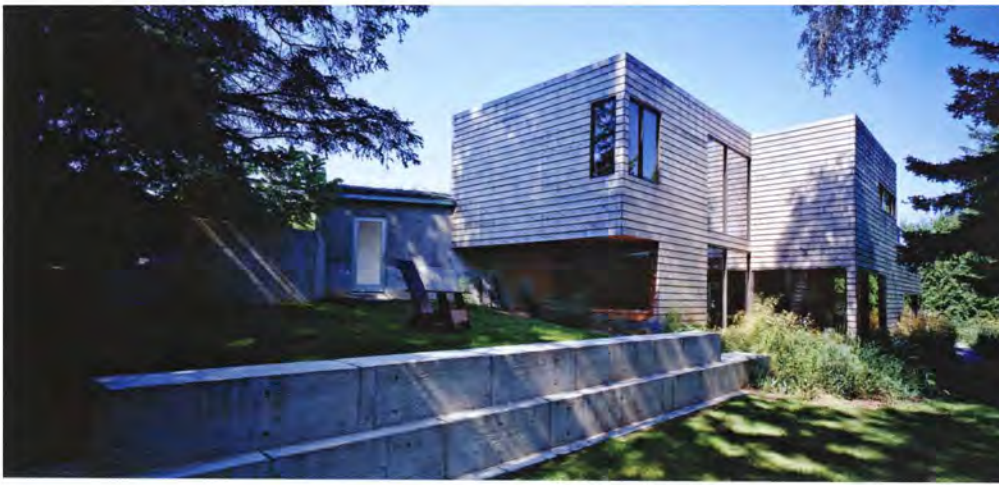
LEFT THE CEDAR-CLAD SOUTH ELEVATION IS AN ABRUPT CONTRAST TO THE CONCRETE AND STUCCO DEFINING THE NORTH ELEVATION OF THE HOME.
