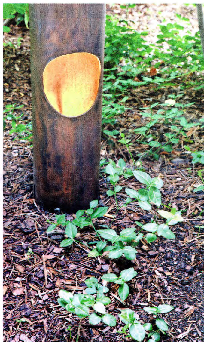
As the building would be used at all hours, the outdoor lighting was essential for safety reasons. The creative solution was to use thick-walled pipes that pop up from the greenery like rusty periscopes.
